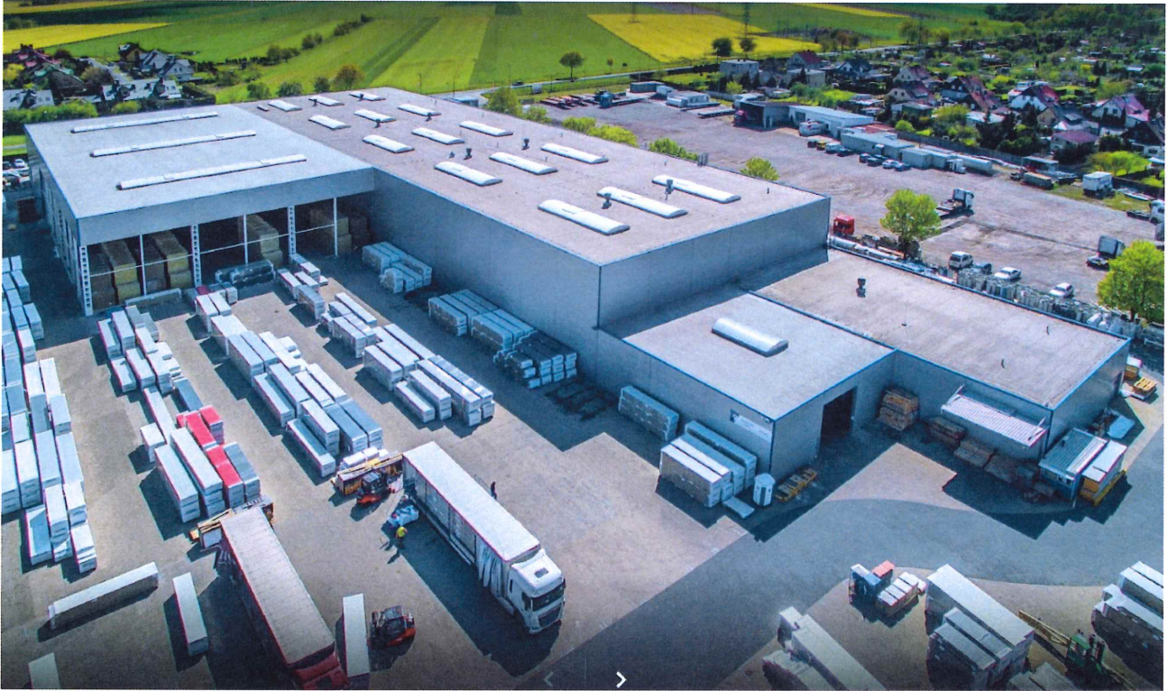
Figure 1. A view of the ARPANEL production hall in Strzelce Opolskie (Poland).
