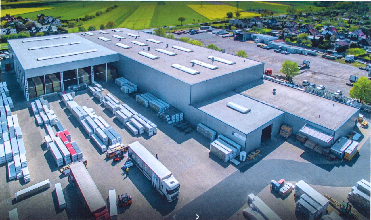
Figure 1. A view of the ARPANEL production hall in Strzelce Opolskie (Poland).
